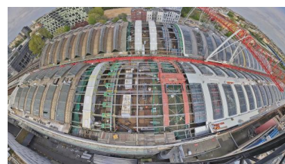
Das Dachpanorama der Station (April 2024) [Quelle: DB Engineering & Consulting GmbH/Marius Müller]
